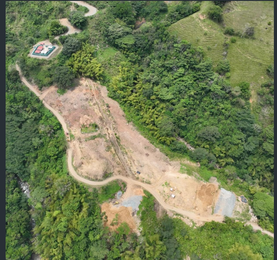
Earthworks are advancing at the plant site
