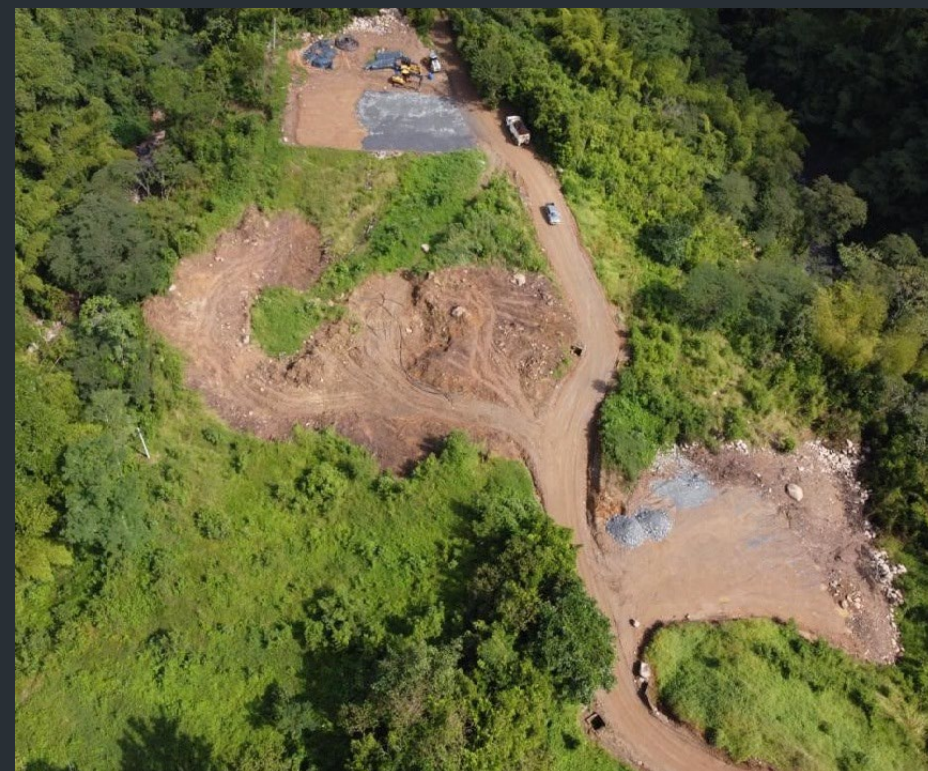
Earthworks have commenced at plant site
